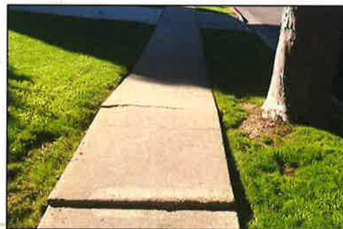
Figure 2: Uplifted Sidewalk
