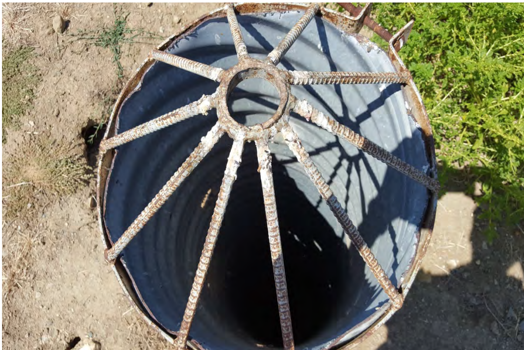
Photo 18. Interior View of Metal Drainage Unit.
