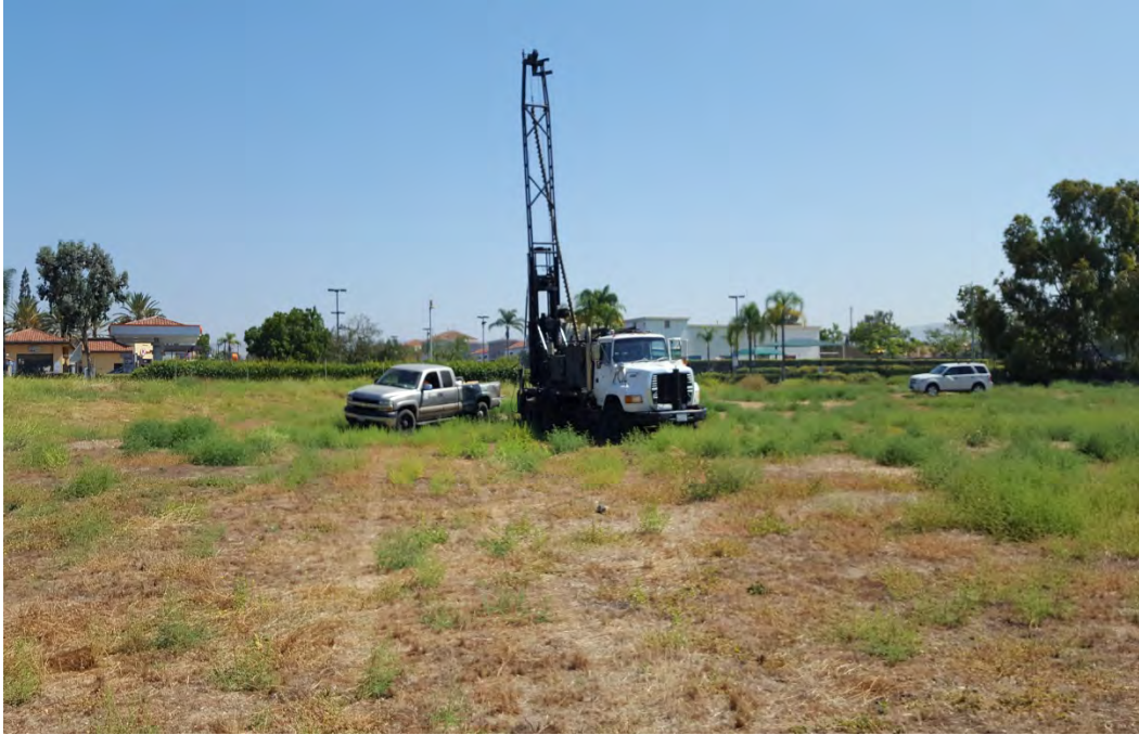
Photo 15. Drill Rig for Collection of Geotechnical Soil Samples by Associated Soils Engineering.
